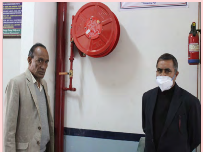
District Fire Officer during Inspection at School Complex
